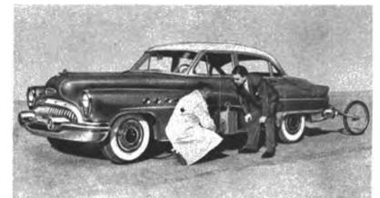
"I was impressed—as I guess every visitor must be—by the test cars that have something resembling a bicycle wheel attached. This 'fifth wheel' is a device for measuring speed and distance with unusual accuracy. On one trip around in a '53 Roadmaster, we found we'd made 17.2 miles on one gallon of gas."
